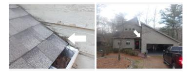
Kickout flashing, also known as diverter flashing, is a special type of flashing that diverts rainwater away from the exterior cladding/siding and into the gutter.
