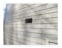
Suggest that additional vents be installed to allow for cross ventilation.
