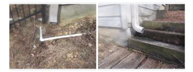
Outlet points need to be located to verify that they are free flowing to daylight and facilitate the discharge and run off of water at least 6' from the foundation.
