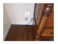
No ceiling light fixture or switch controlled wall outlet for sleeping area.
