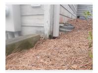
Entry point for buried leader at front corner was not visible and is disconnected from the downspout.
