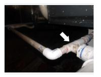
No condensate overflow pan and float switch.
