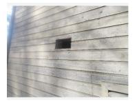
Suggest that additional vents be installed to allow for cross ventilation.
