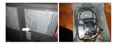
Oversized breaker. Data plate specifies a maximum over current protection of 20amps.
