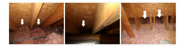
No roof vents for attic area under front shed roof.
