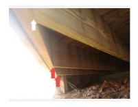
Deck is in contact with the ground. Deck materials need to have clearance above grade.
