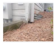
Entry point for buried leader at front corner was not visible and is disconnected from the downspout.
