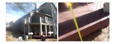
Several missing joist hangers at rear of deck.
