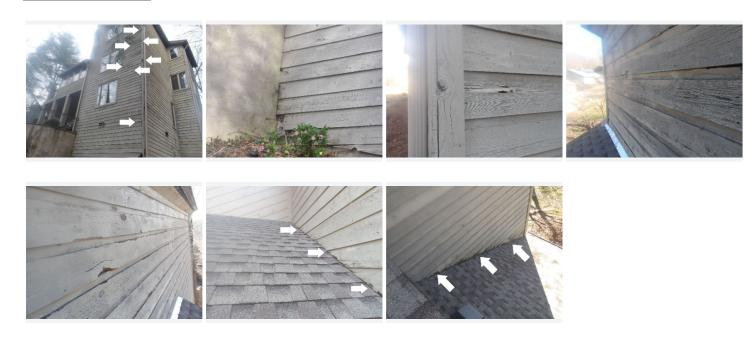
All grade and ground cover need to be pulled away from contact with the wood siding. Siding clearance should be between 6"-8" from grade.
