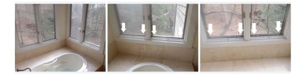
Window around tub could not be opened do to missing crank handles.
