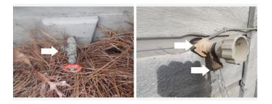
Leak at valve stem for hose bib under electric meter when valve is open.
