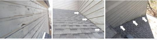
All grade and ground cover need to be pulled away from contact with the wood siding. Siding clearance should be between 6"-8" from grade.
